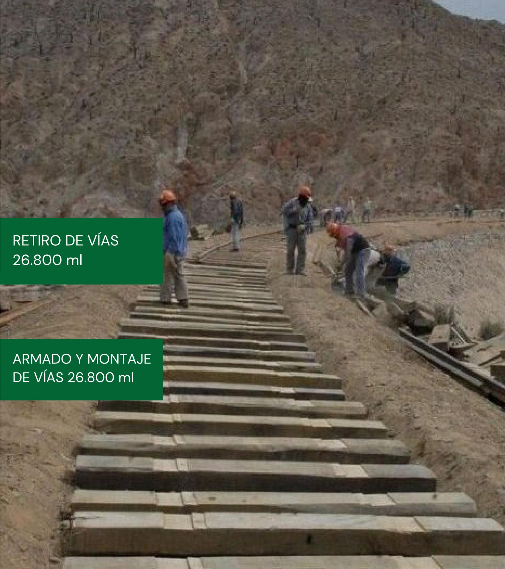
A photograph showing a railway construction site in a mountainous, arid region. Several workers wearing hard hats and work clothes are visible, engaged in the process of removing old tracks. The ground is covered with gravel and dirt, and the background shows steep, rocky hills.
